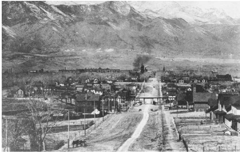
Colorado Springs, Colorado from around the time Tesla was there
